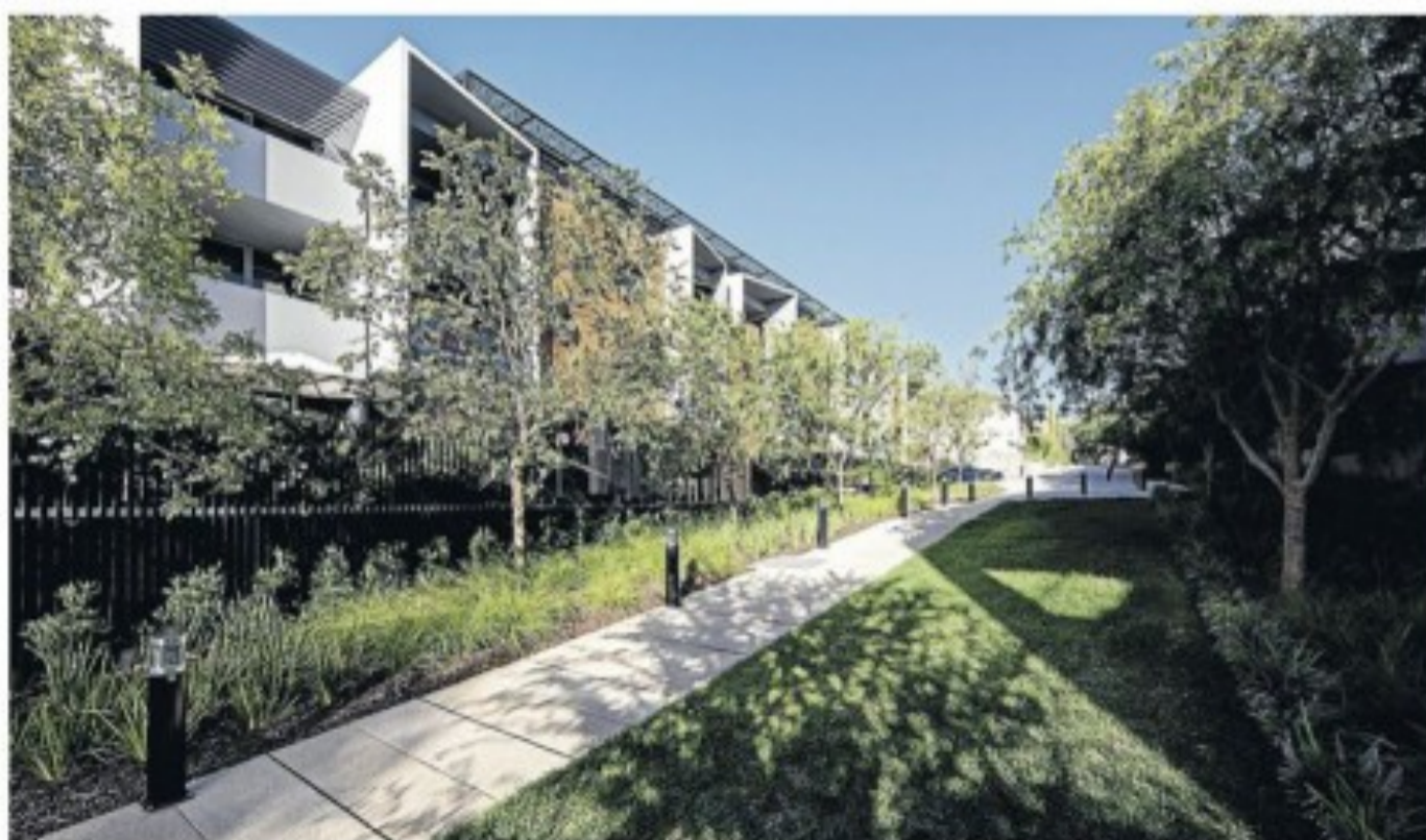
Green corridor: The Malvern Hill development features a central landscaped courtyard garden.
